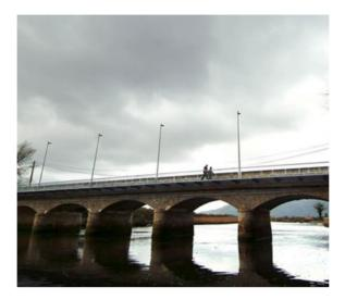
The Ponteceso Bridge over the River Anllóns was built between 1868 and 1879, and allows the AC-430 road and pedestrian traffic to access the village of Ponteceso. The Anllóns River at Ponteceso is close to its flow into the Atlantic Ocean, thus influenced by tidal sea level variations with low tide water levels reaching the upper part of the foundations, and high tides rising up to 2.15m over the aforementioned level.
